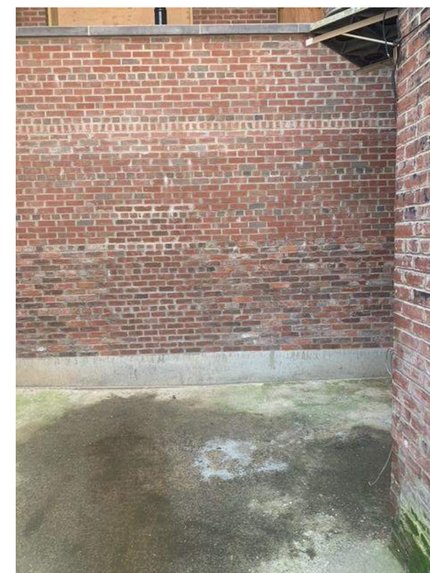
SOUTH PROPERTY LINE AT NEW DEVELOPMENT WALL
